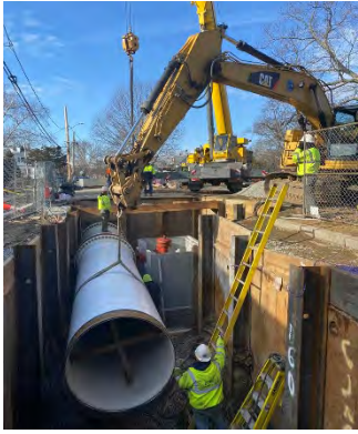
WASM 3 – pipe replacement
