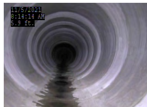
WASM 3 - cement-mortar lined steel pipe
